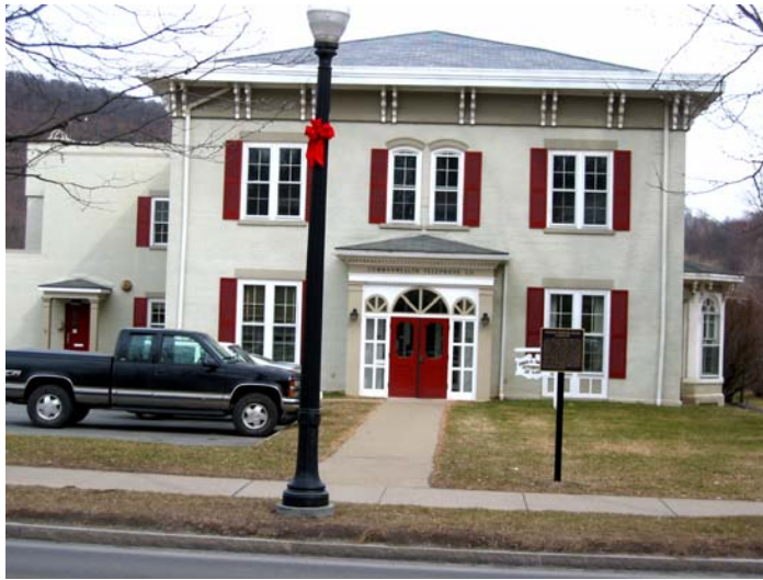
Historic York Avenue Structure Now Occupied by Frontier Communications
