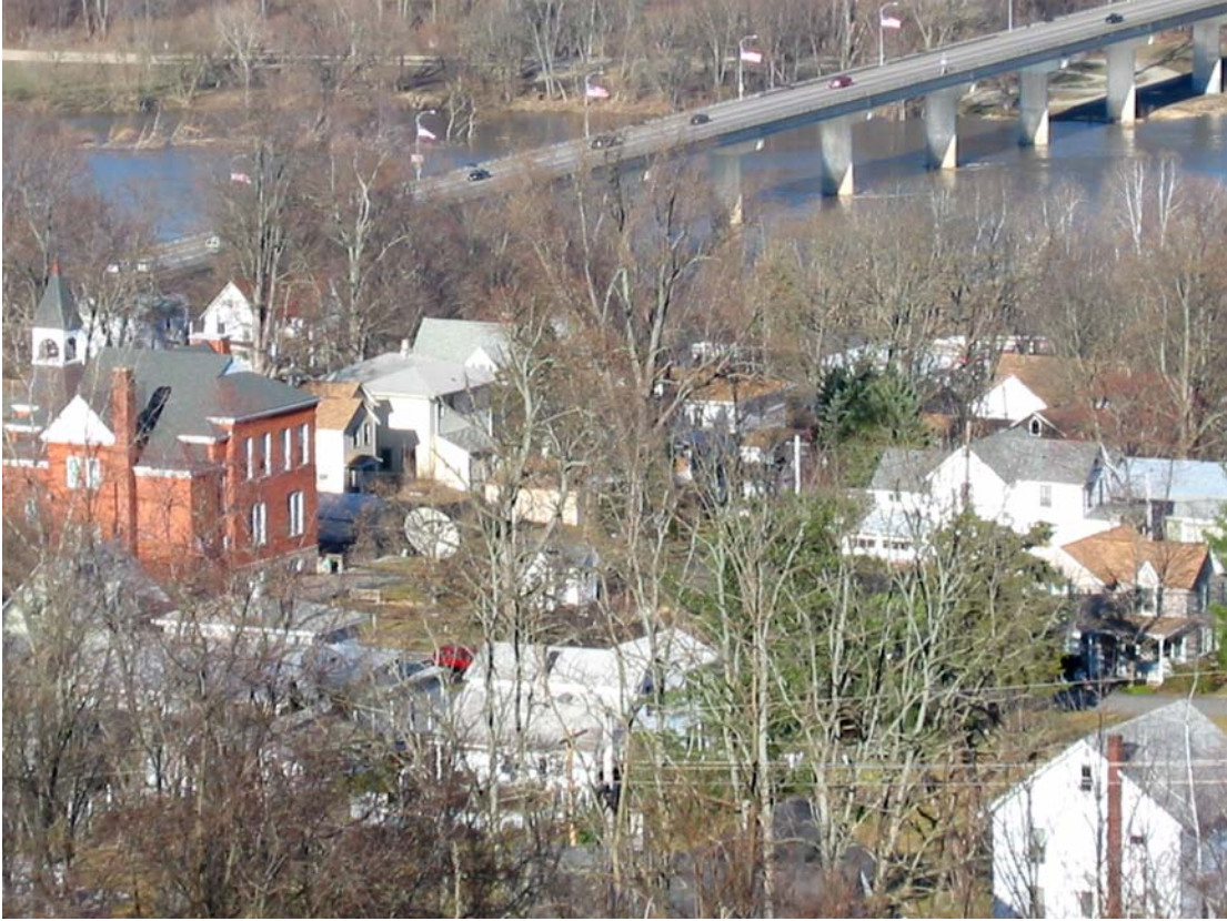
View of Veterans Memorial Bridge from Bridge Street Hill Rd.
