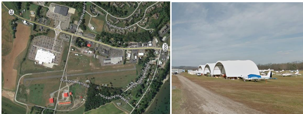
Figure 18: Views of Skyhaven Airport
