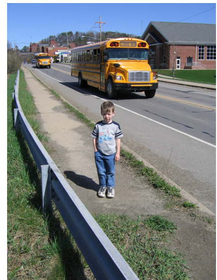
The sidewalk ends abruptly with no crosswalk in front of Mansfield High School.
