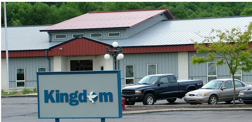
Growth at Kingdom, Inc., contributes to traffic at the intersection of Route 6 and Lambs Creek Road.
