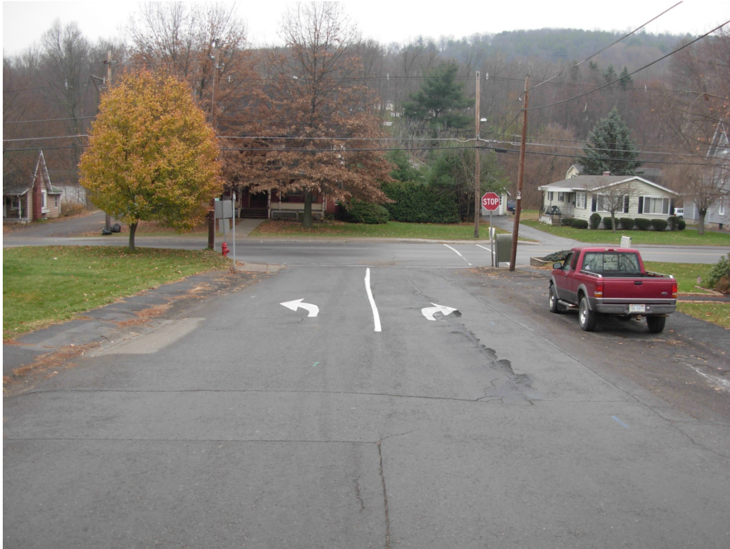
Eastbound King Street Approach
