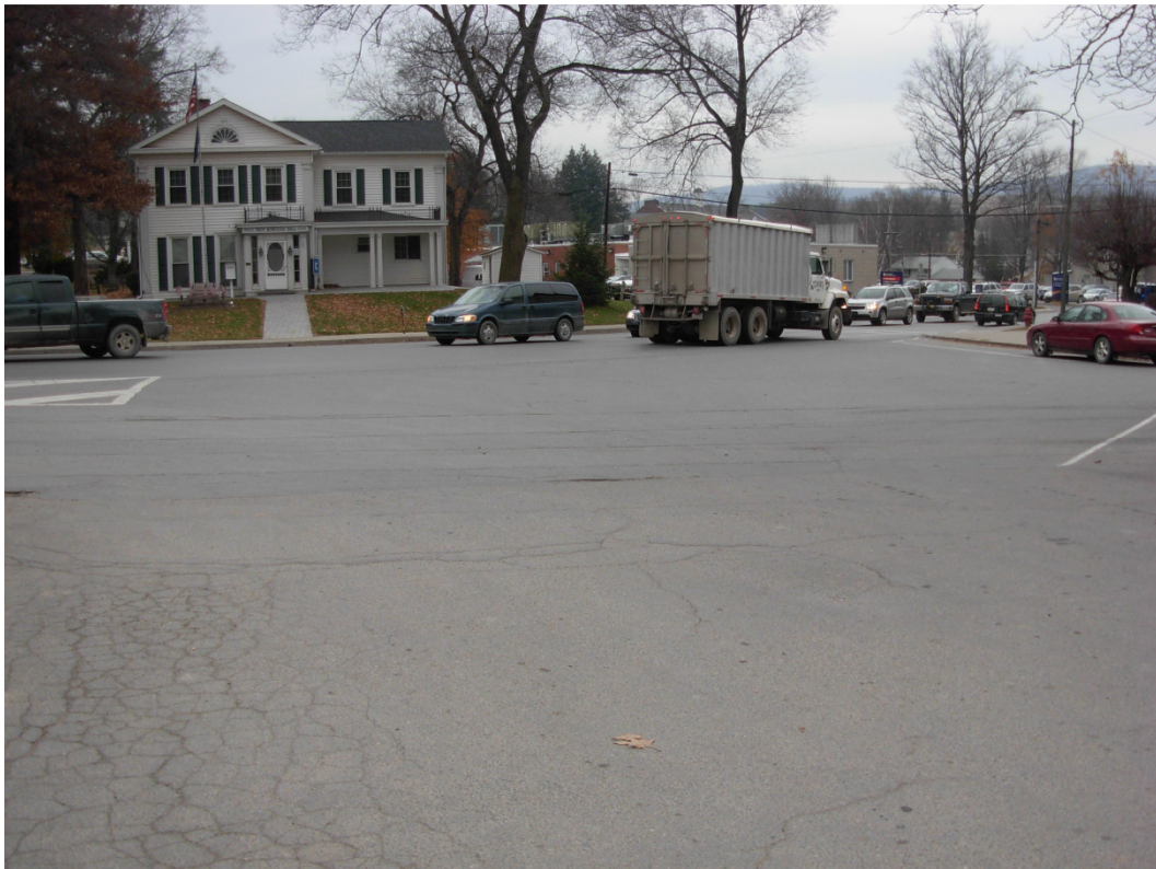
Northbound Parking Lot Access Approach
