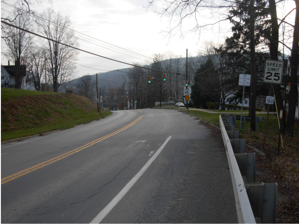
US 6 Eastbound Approach (First Light)
