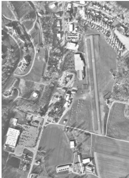
Figure 7: Aerial View of Sky Haven Airport
