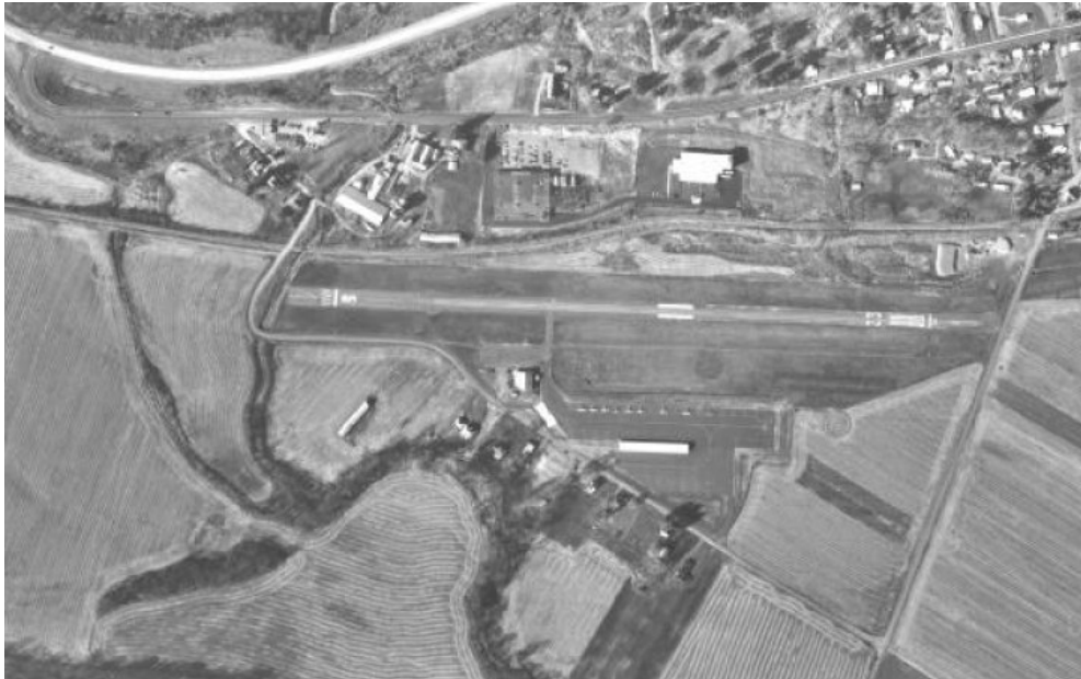
Figure 5: Aerial View of the Bradford County Airport
